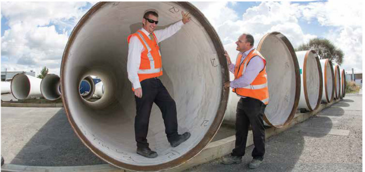
Project manager David Moore and site supervisor Craig Matthewson inspect some of the pipes being used for the Hunua 4 Watermain project. This 32-kilometre pipeline will ultimately connect the reservoirs at Redoubt Road in Manukau to those in Khyber Pass, Grafton. The large-diameter pipe – up to 1.9 metres – will service all communities along the route.
